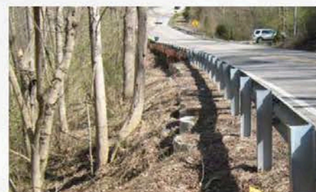
Completed Landslide project on Roundbottom Road
