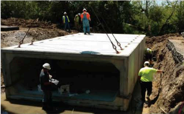
Taylor Pike Bridge Under Construction
