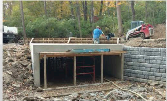
No. 9 Road Bridge Under Construction
