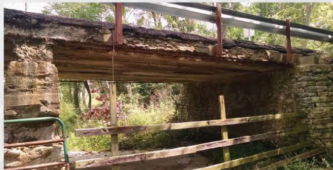
Existing Johnson Road Bridge
