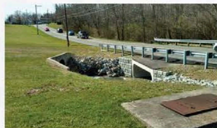
Woodville Pike reconstruction project
