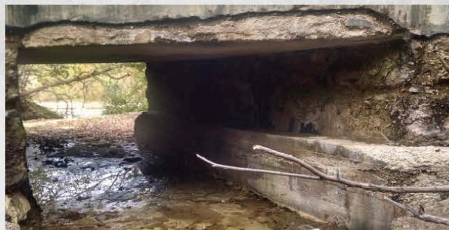
Existing Shinkles Ridge Bridge
