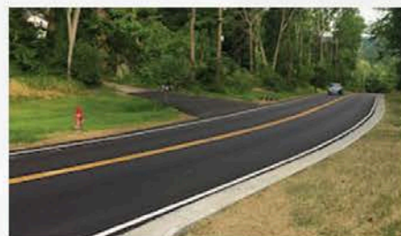
Completed work on Branch Hill Guinea
