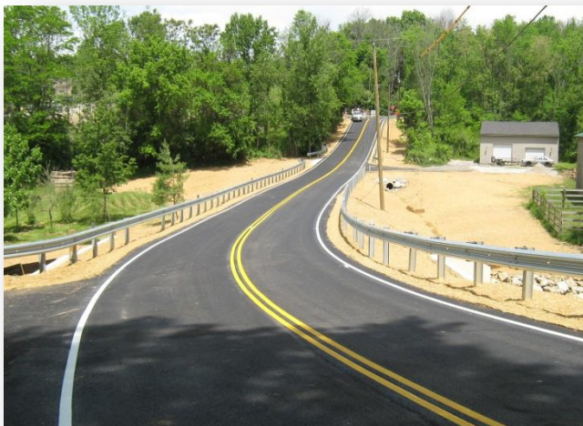
Mt. Pisgah Road and bridge improvements completed in 2015.
