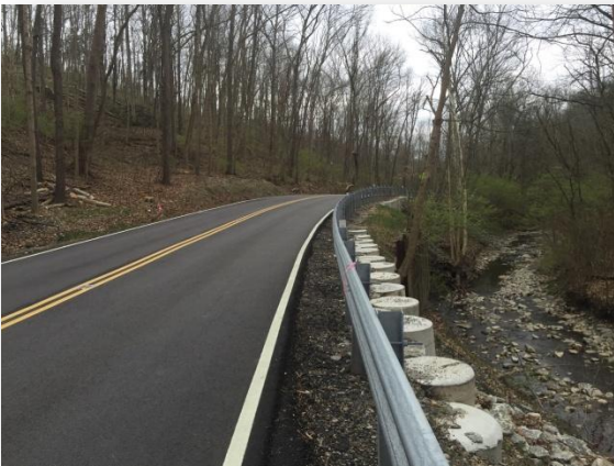
Completed Landslide project on Wolfpen-Pleasant Hill Road in 2015
